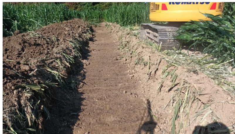
Plate 6: Trench T6, looking W
