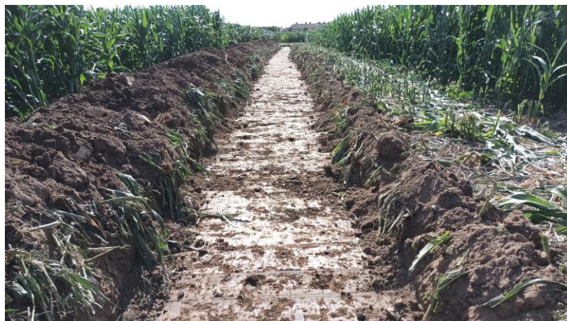
Plate 3: Trench T3, looking SE
